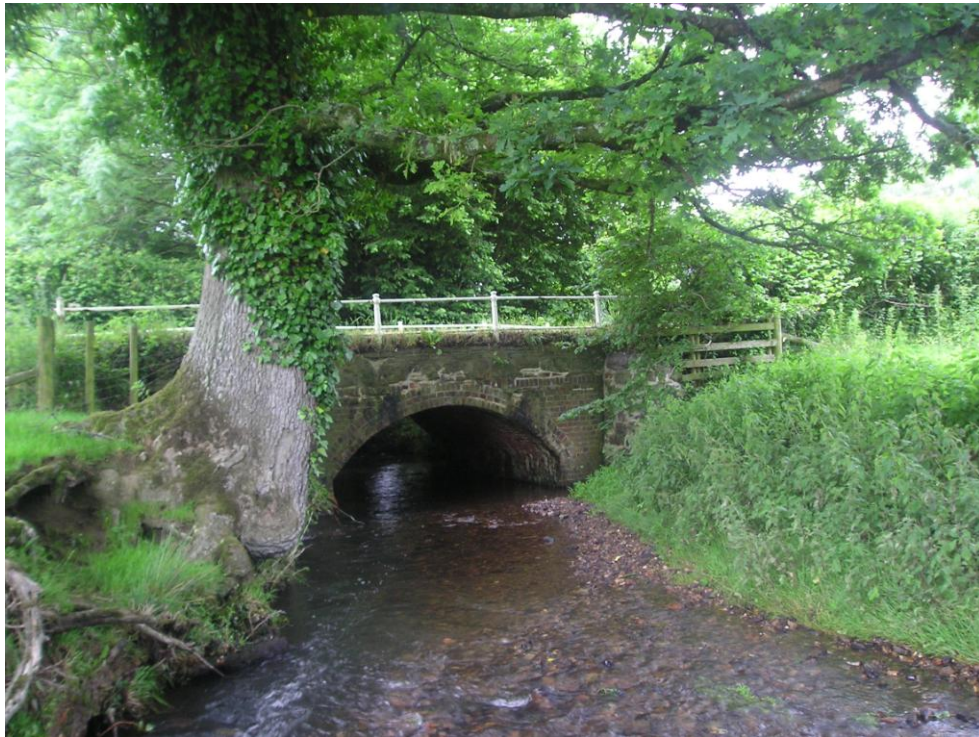
Shedrick Bridge, Wheel House Lane
